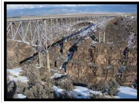
Rio Grande Gorge Bridge near Taos, New Mexico
